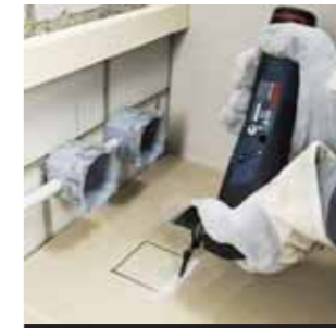
Plunge cuts in dry wall, e.g. for power sockets
