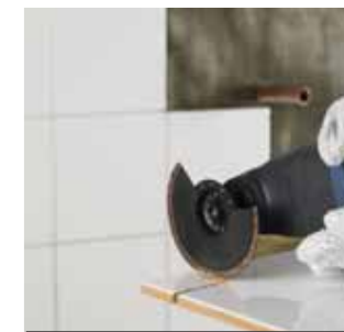
Cutting of soft tiles, e.g. small cut-outs in soft wall tiles
