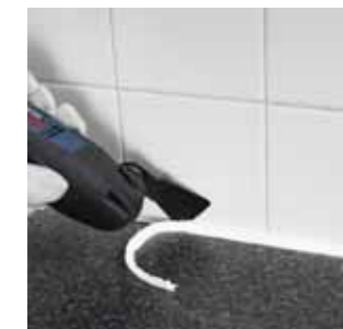
Scraping, e.g. removal of caulking seams
