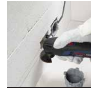
Cutting slots in porous concrete, e.g. for installing tubes and cables
