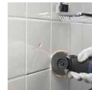
Reaming seams between wall or floor tiles, e.g. to remove broken tiles
