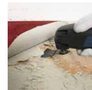
Scraping, e.g. remove glue from surfaces after carpet removal
