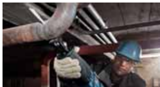
Cutting metal pipes
